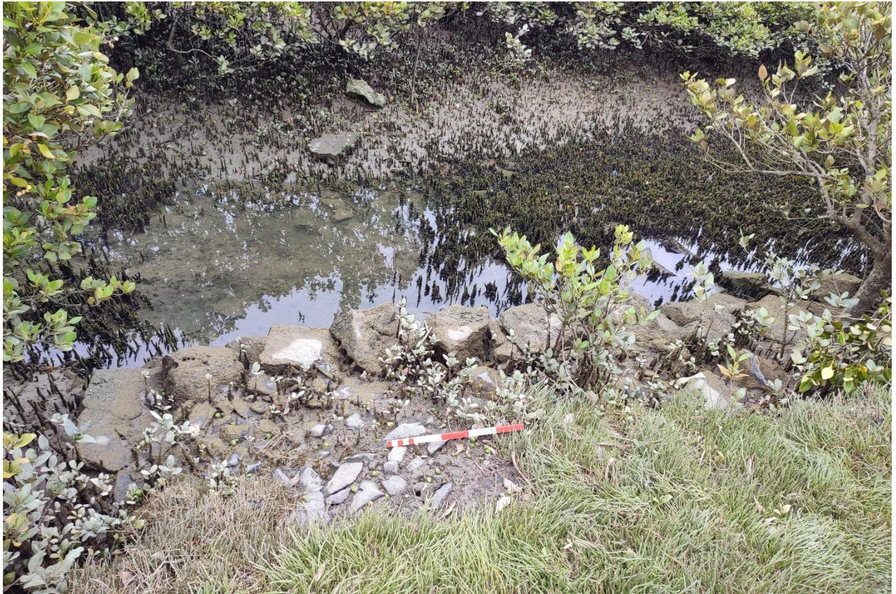
Figure 4-5 View west from northern quay showing dry stone construction. Photo scale = 0.5m.
